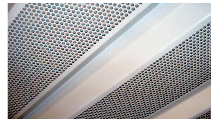
Circular perforations within the trough of the liner profile only, providing an open area of 22%.
