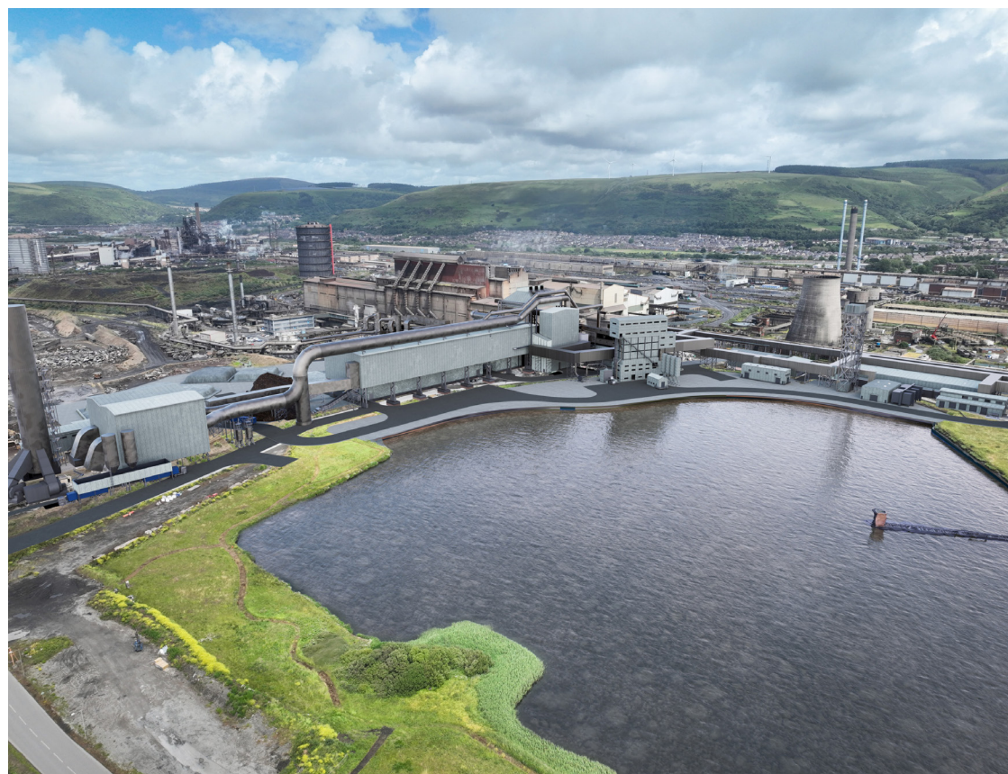
Glimpse into the future... How the EAF building will look once completed
