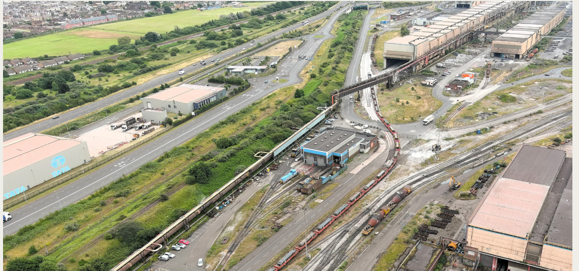
The snakelike 25 wagons carrying around 2.3KT of slab into Port Talbot in what will be daily deliveries for the next three years until the EAF is up and running
