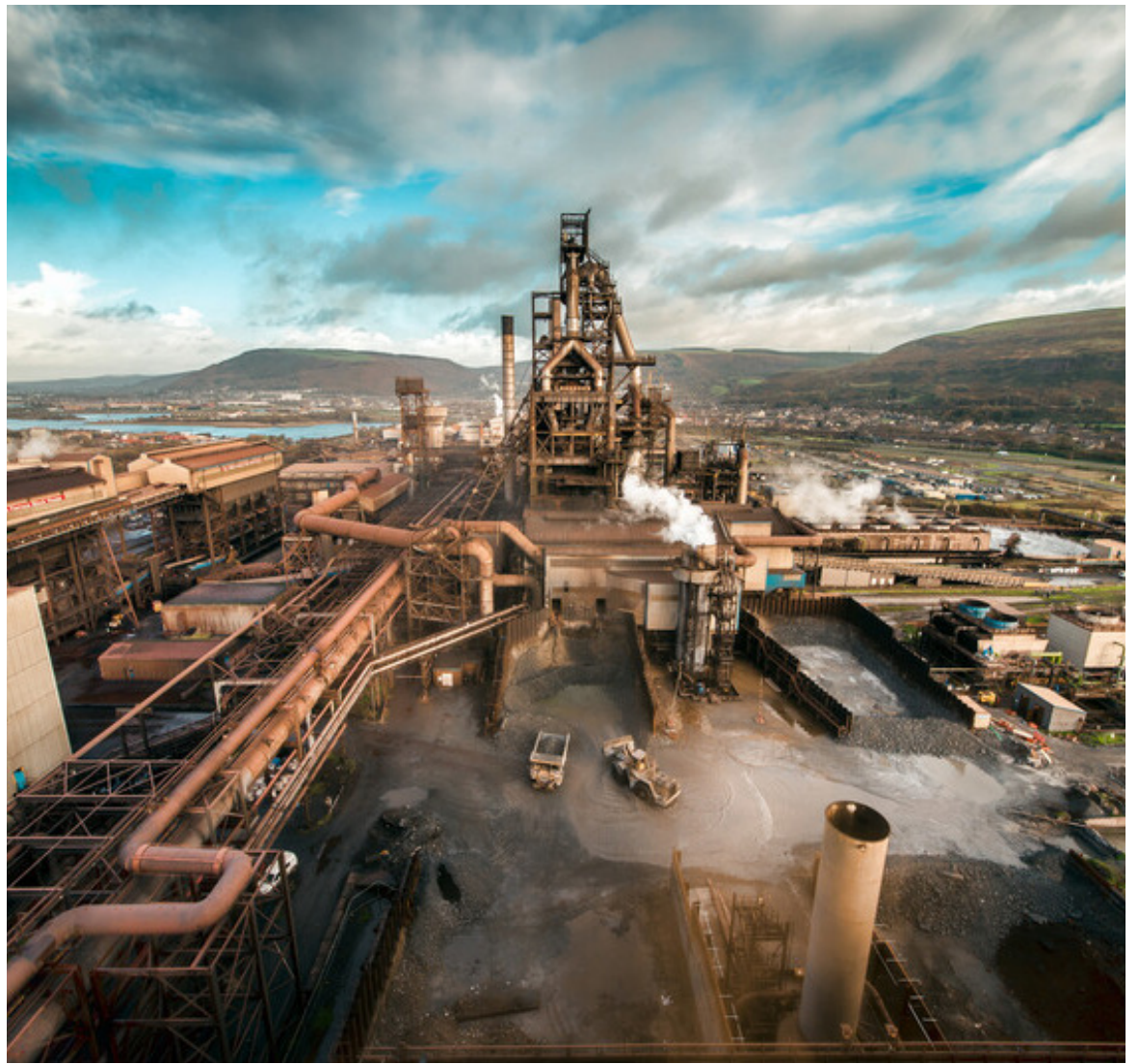
Aerial View of Blast Furnace 4
