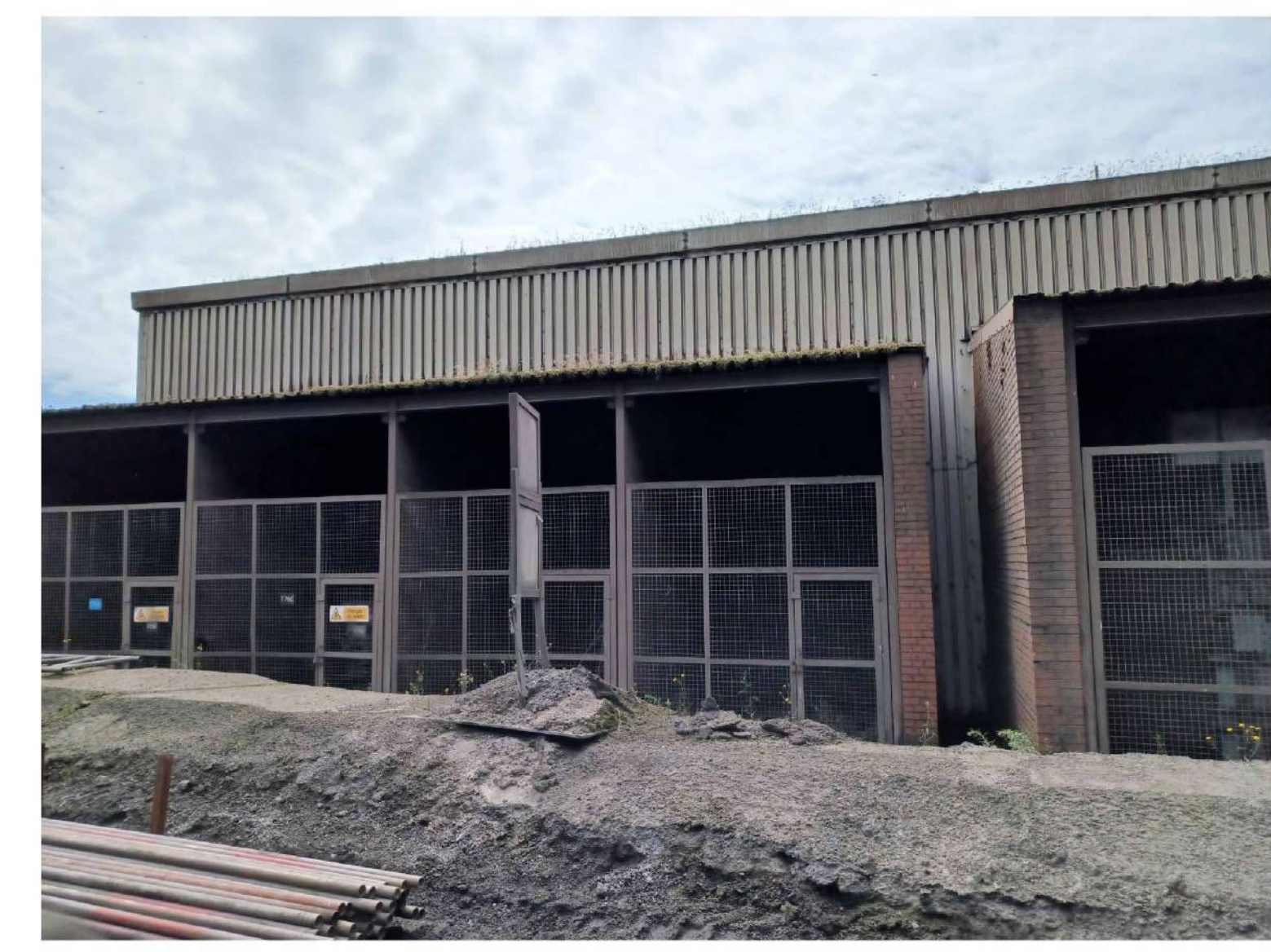
Photo 2 - Existing Compressor House With MCC Room
