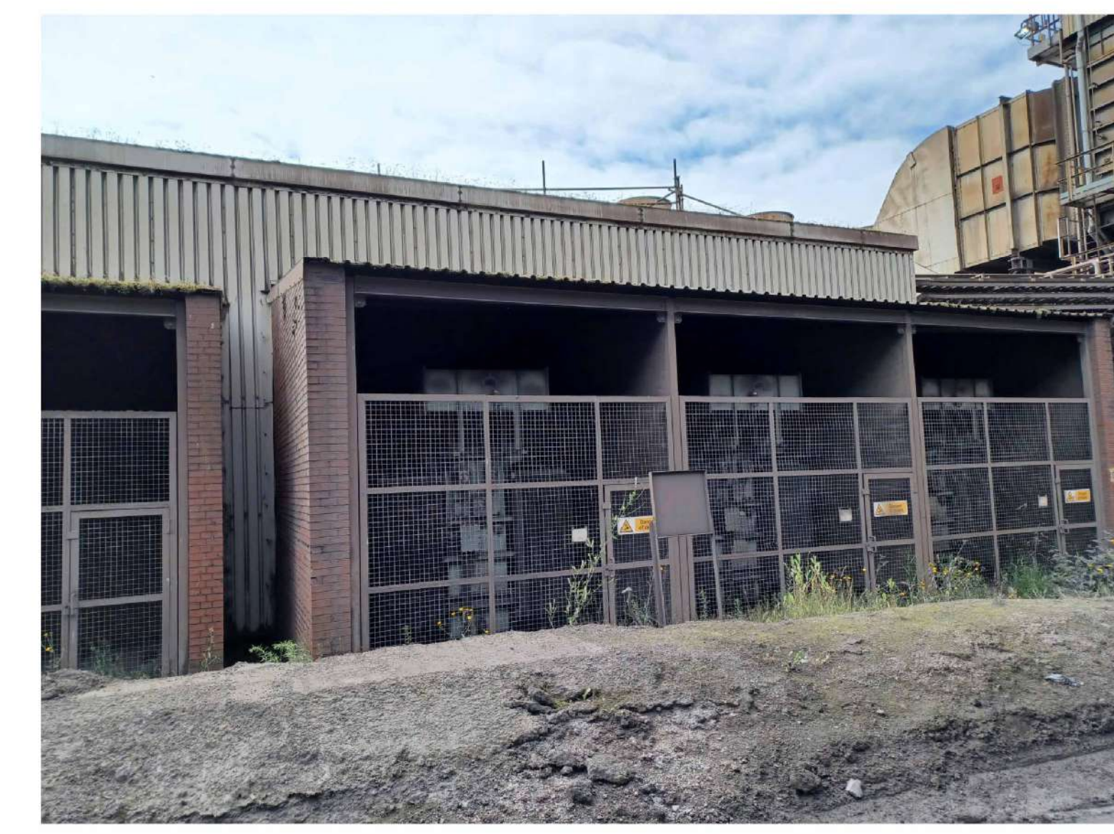
Photo 3 - Existing Compressor House With MCC Room
