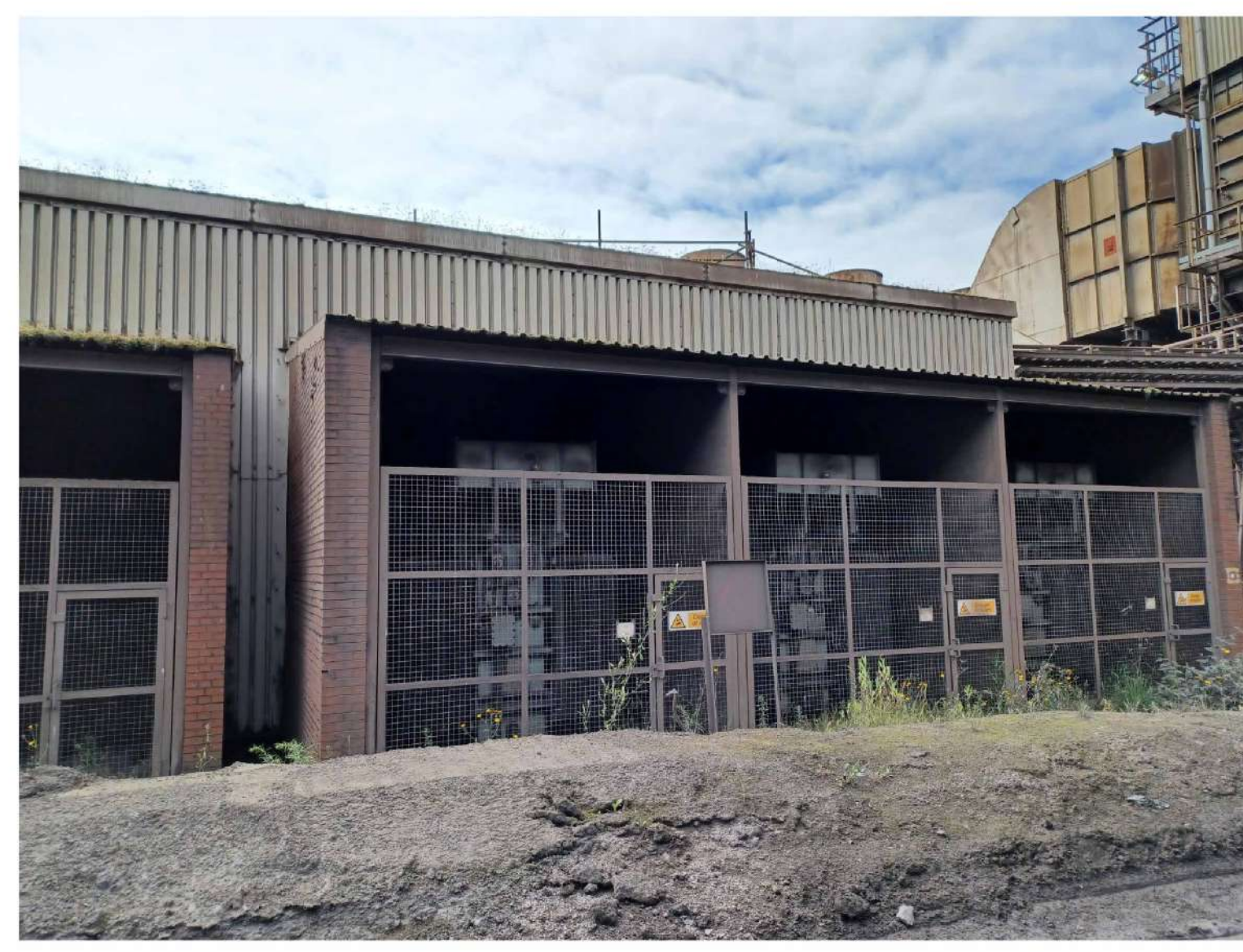
Photo 1 - Existing Compressor House With MCC Room
