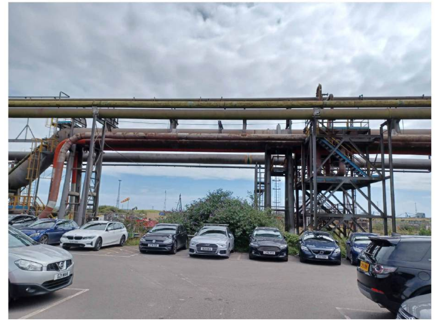
Photo 4 - BF Gas Pipe Rack (Partially Removed)
