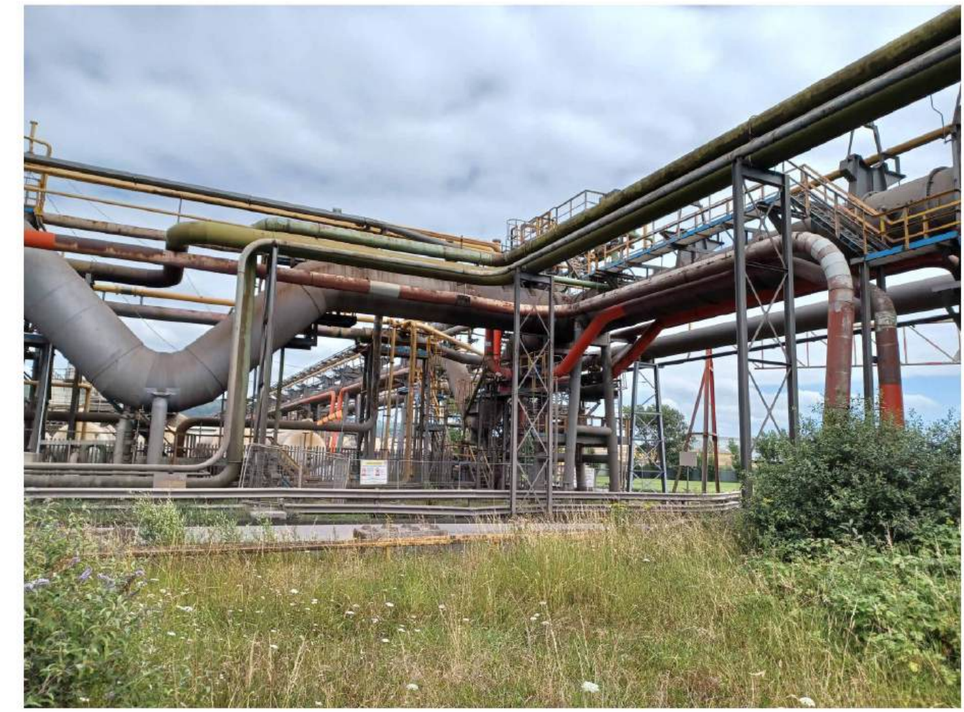
Photo 3 - BF Gas Pipe Rack (Partially Removed)
