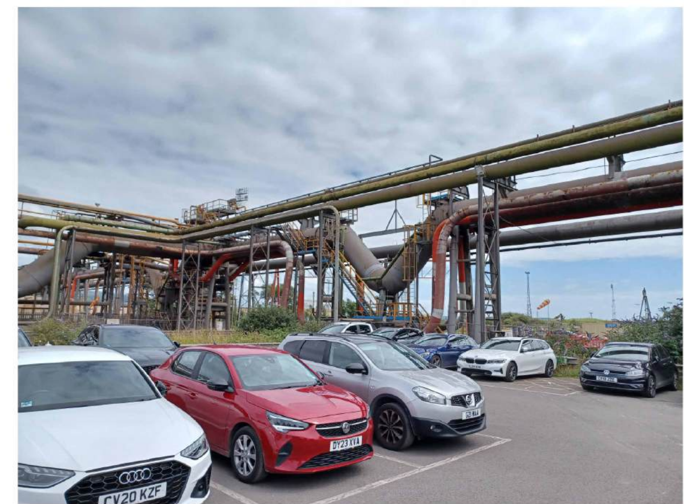
Photo 2 - BF Gas Pipe Rack (Partially Removed)
