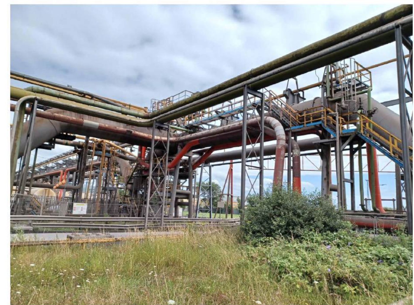
Photo 1 - BF Gas Pipe Rack (Partially Removed)
