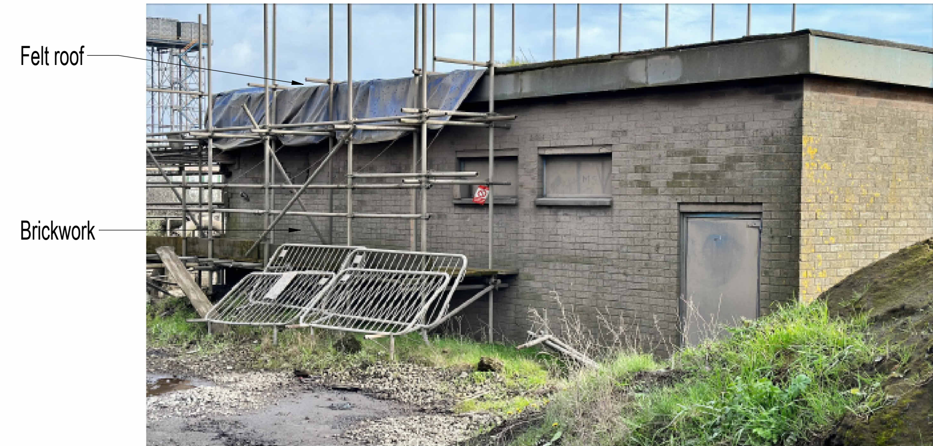
Photo 2 - Existing Pump House
