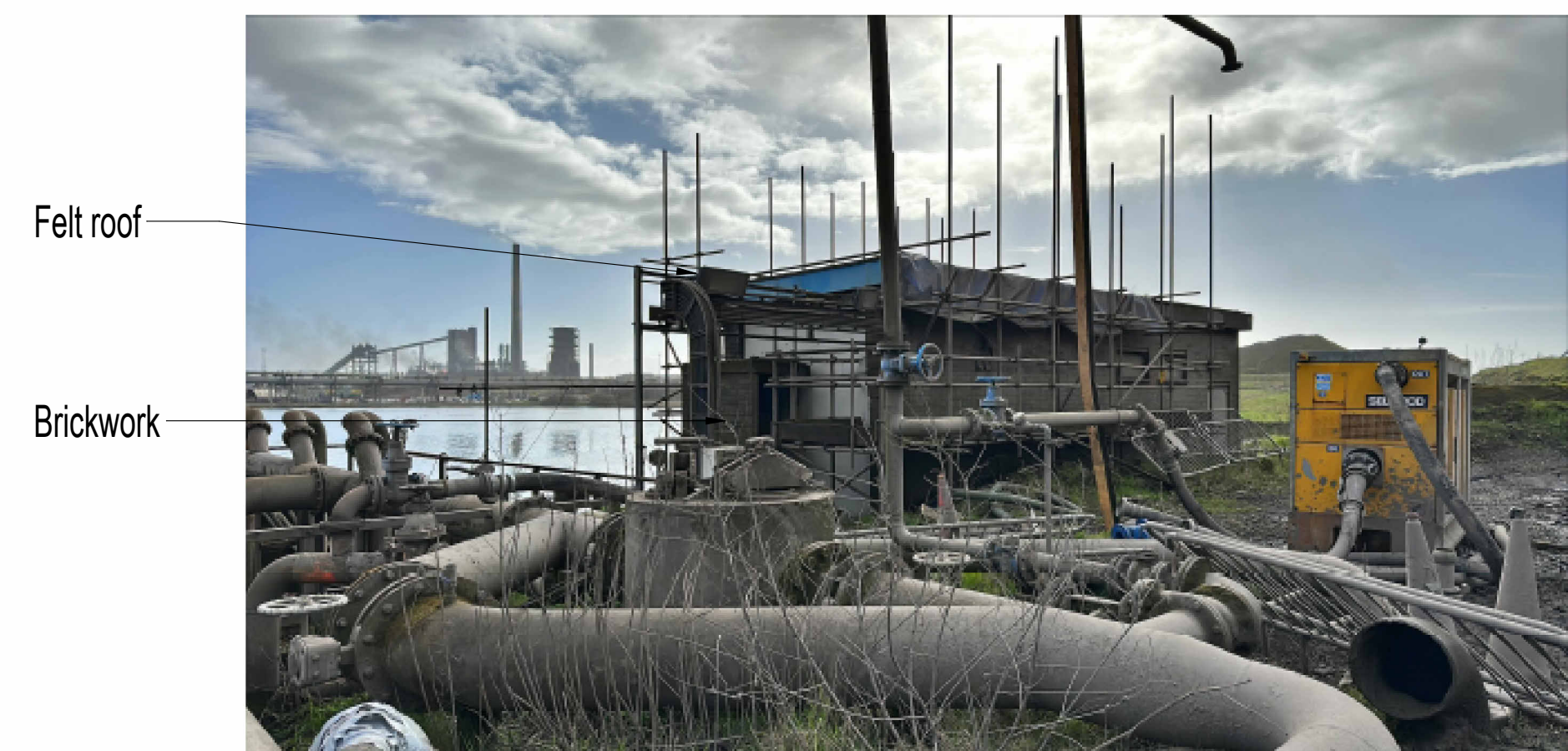
Photo 3 - Existing Pump House
